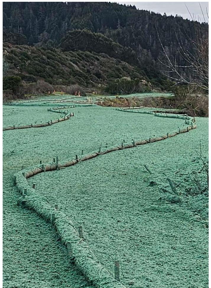
View of the January 26 th , 2026 hydroseed application containing a sterile wheatgrass mix to assist in erosion control.
